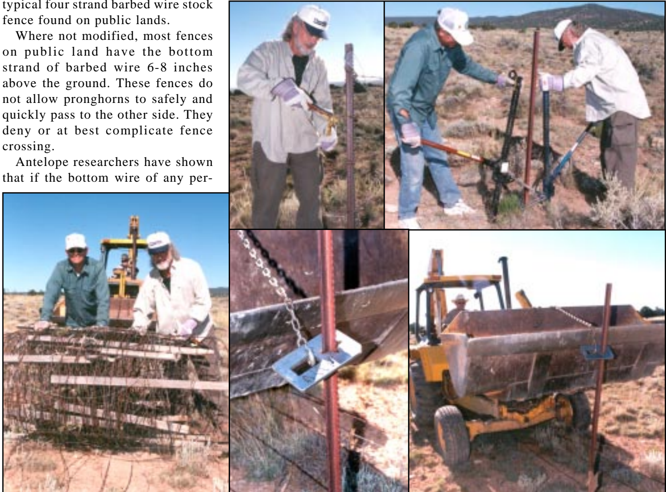
Clockwise from above: Lee Kohlhasse of Mesa and John Sampanes of Paradise Valley rolling up a downed fence with stays attached; John easily clips t-post clips with bolt cutters, freeing the wire; Lee and John pulling a stubborn t-post with two high lift jacks and using a special plate that is designed to quickly and easily grip the post and allow them to be "jacked" out of the ground; Another faster method of removing posts utilized a front loader and a logging chain. The plate is dropped over the post with chain attached then pulled from the ground, easily slid out, and deposited into the bucket. (close up center); A two man team can over a mile of fence posts in a little over an hour; Right: A morning's accumulation of fence.
